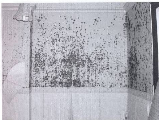
Fig. 1. Mould growth on the dining room walls of the infested property.
